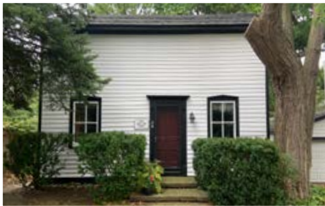
The Michael Quinn House (built in 1855, 38 Burnet Street) exemplifies an early clapboard-covered home with two windows, a centre door, a
