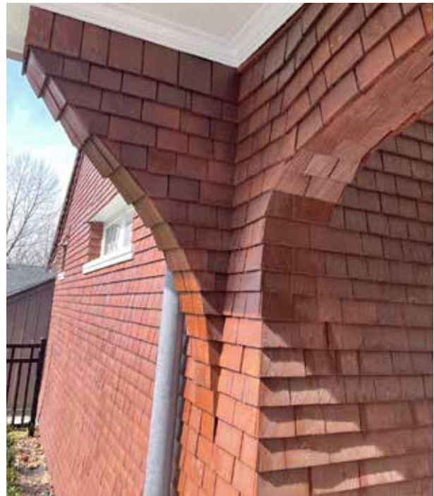
Steam-treated curved cedar siding with lead coated copper downspout
