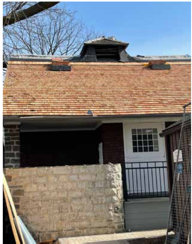
The new roof with the manure pit in the foreground
